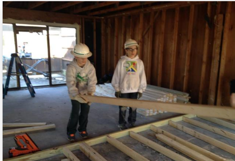
ARC Home Renovation Project (2016)
